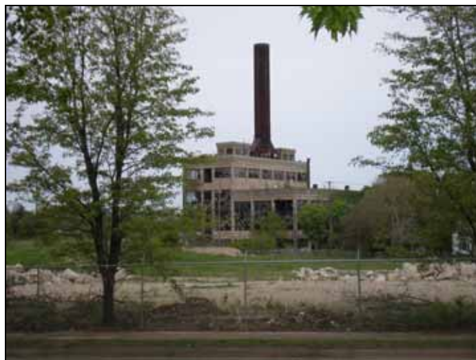
Former power plant, now owned by the City and being demolished.
